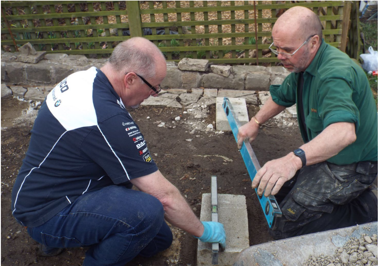
Laying the foundations: Meanwood Men Shed
