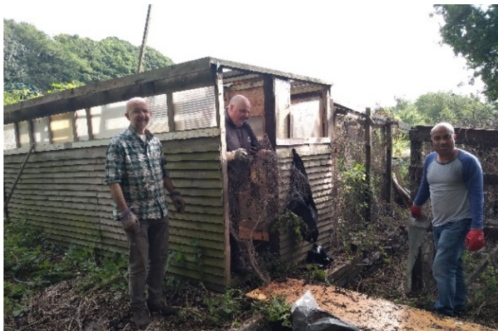
Clearing old buildings to make way for the new
